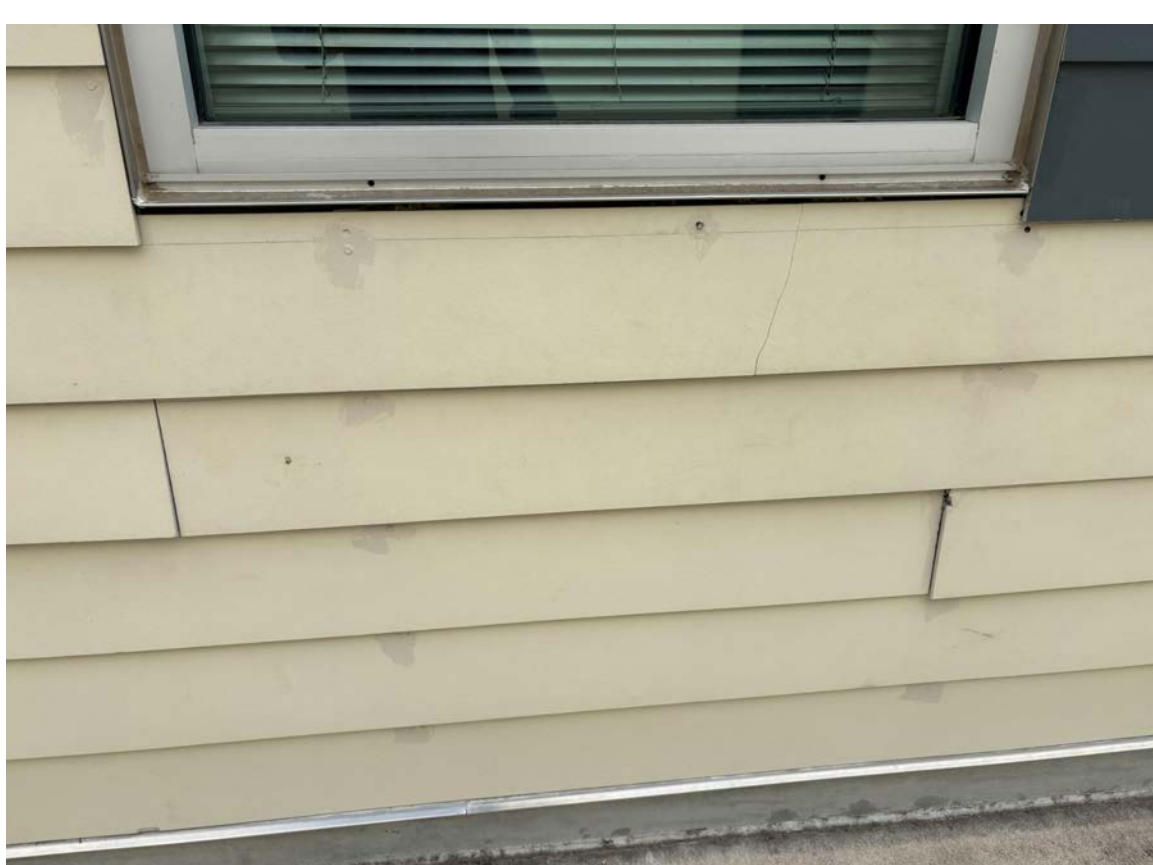
REPLACED DAMAGED AND WARPED SIDING
