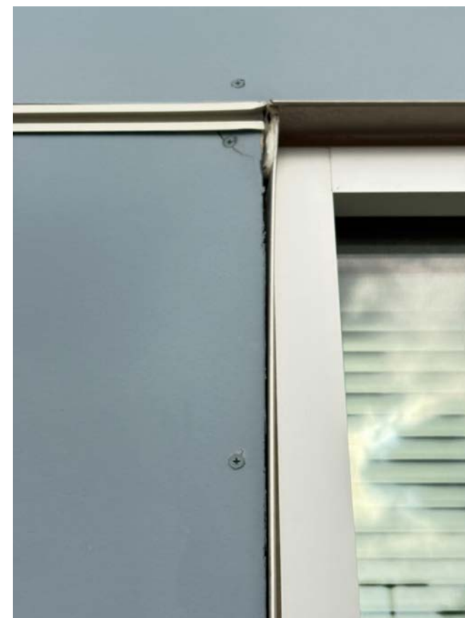
REPLACE DAMAGED SIDING
