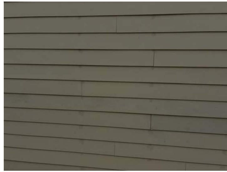
REPLACE DAMAGED SIDING
