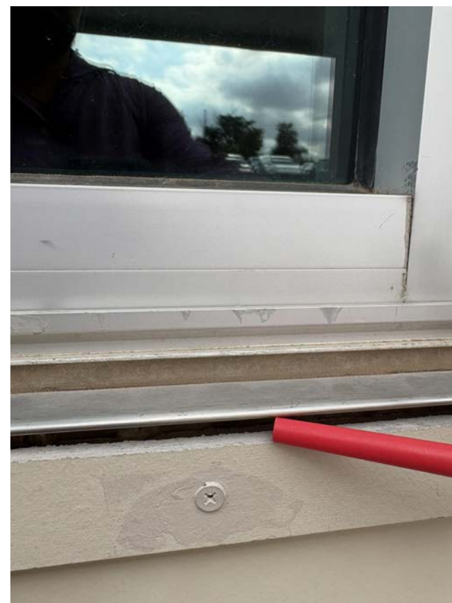
REPLACE DAMAGED SIDING
