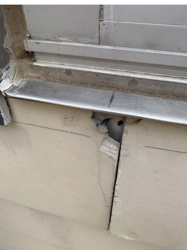
REPLACE DAMAGED SIDING
