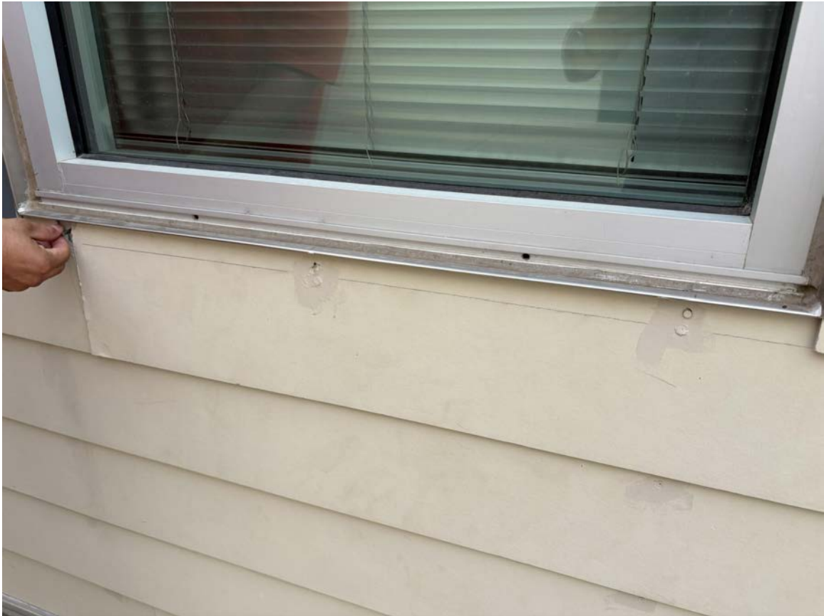
REPLACE DAMAGED SIDING
