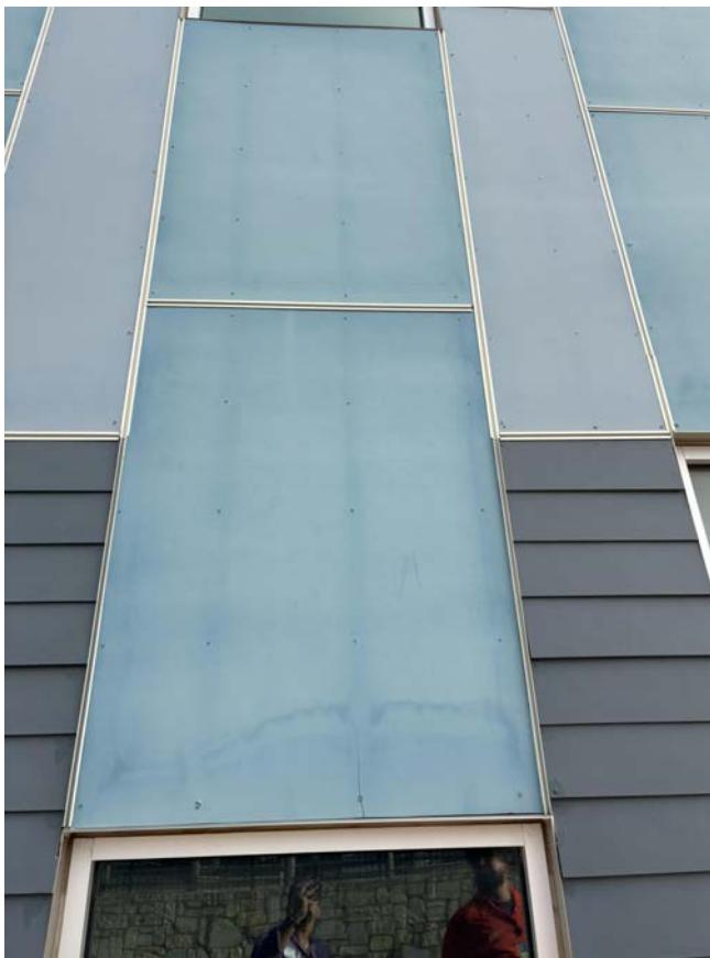
REPLACED DAMAGED SIDING
