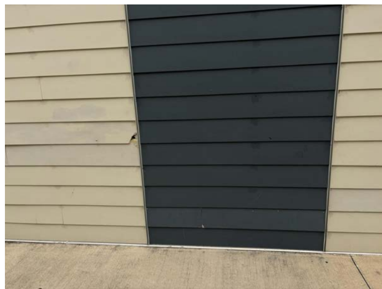
REPLACE DAMAGED SIDING
