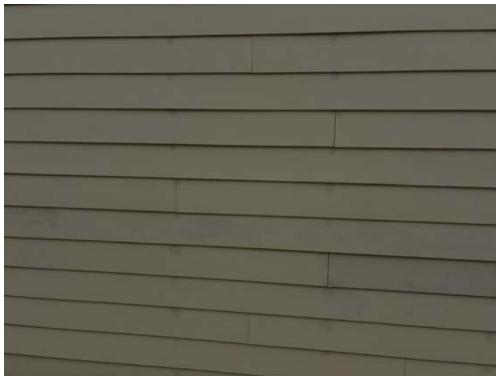
REPLACE DAMAGED SIDING
