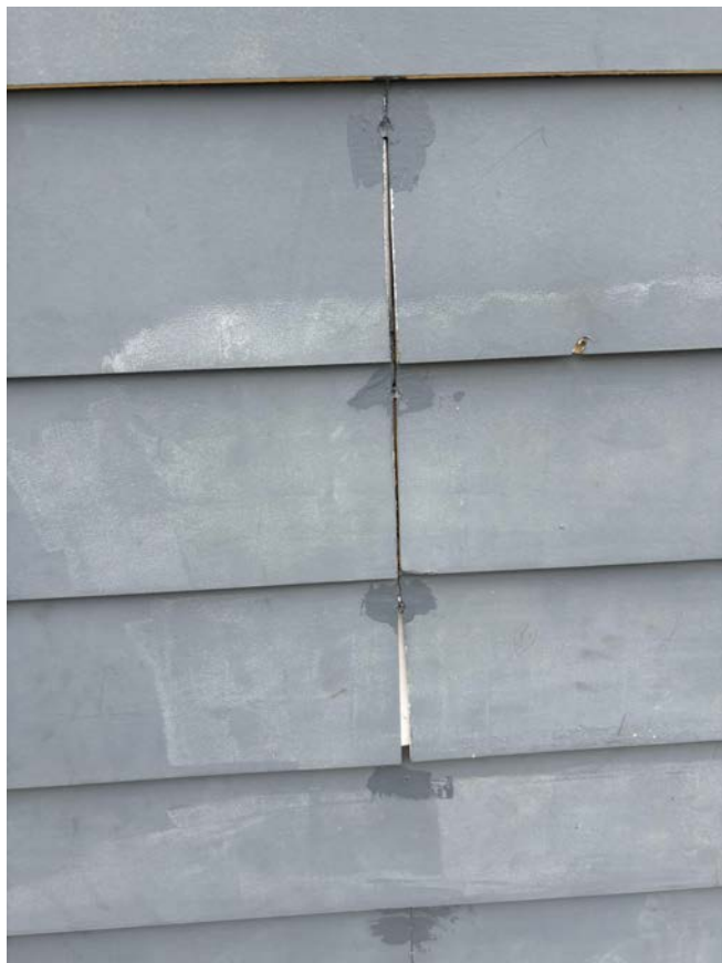
REPLACED DAMAGED SIDING
