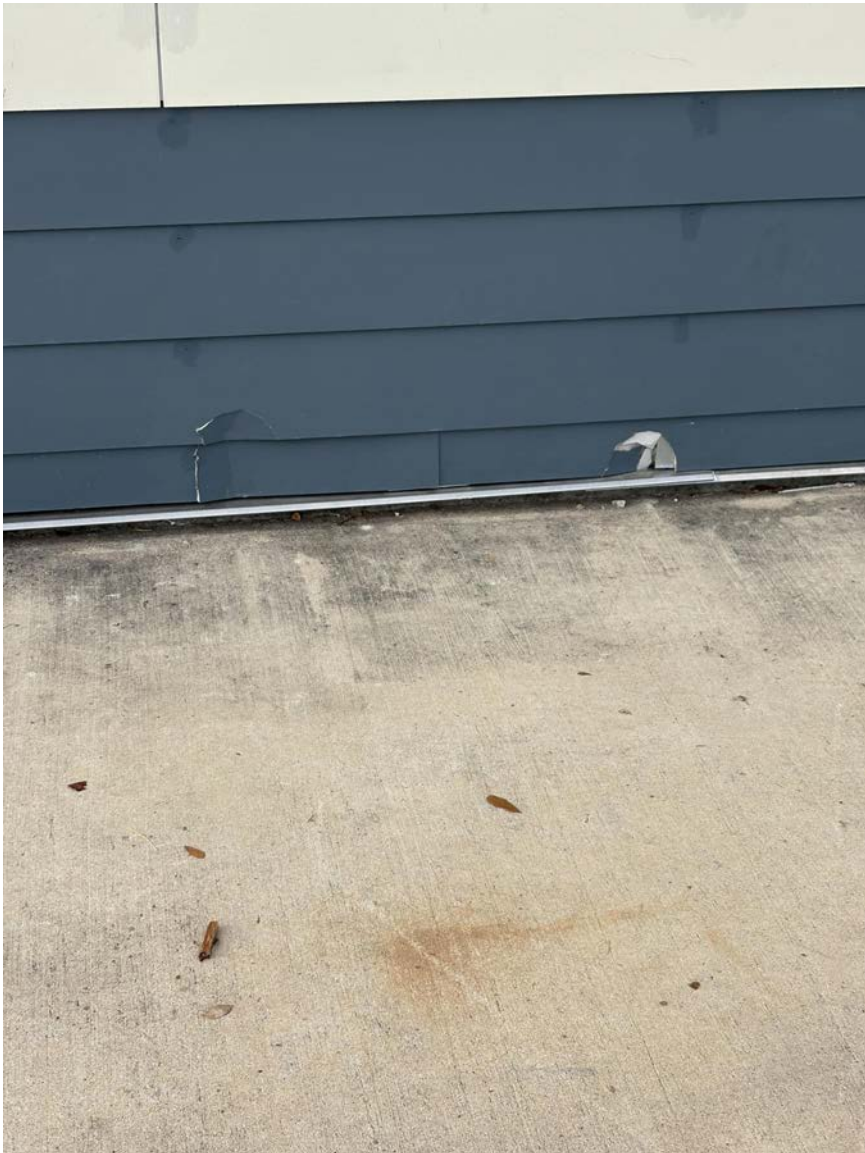
REPLACED DAMAGED SIDING
