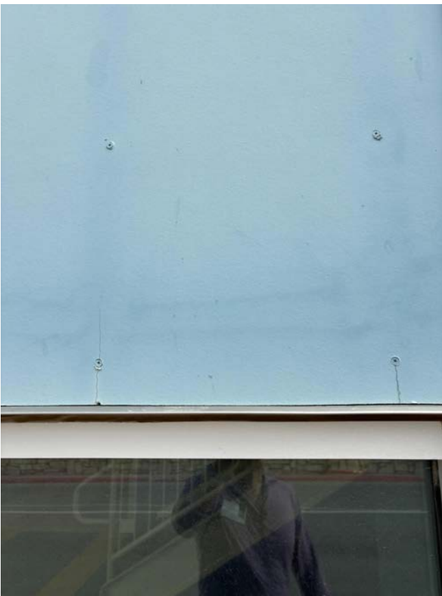
REPLACED DAMAGED SIDING
