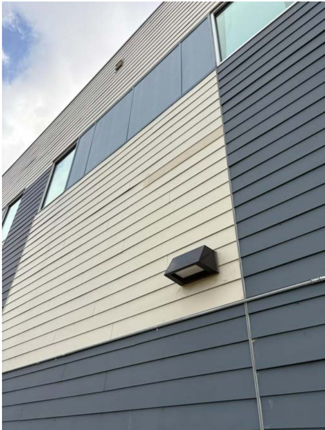
REPLACED DAMAGED AND WARPED SIDING
