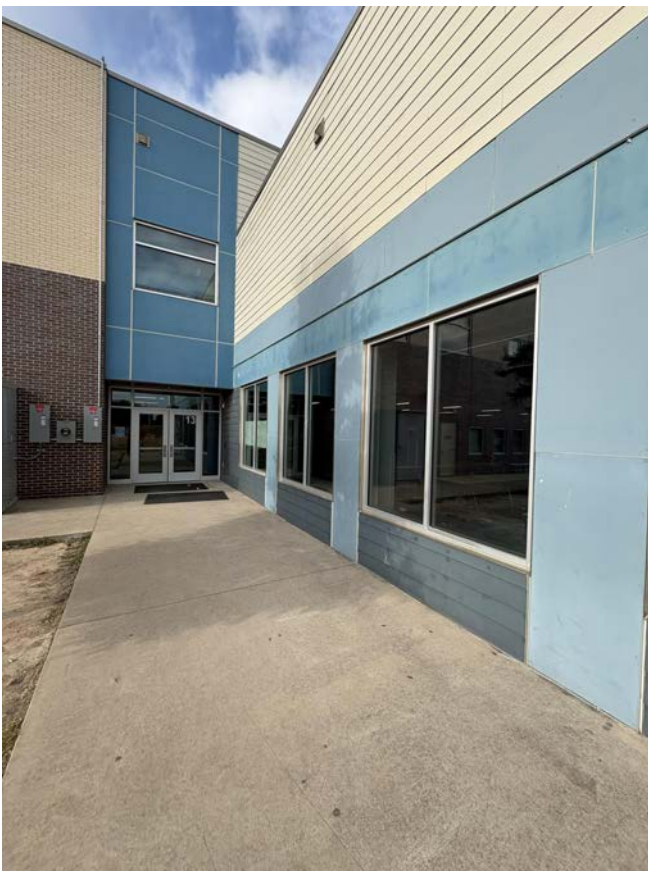
REPLACED DAMAGED AND WARPED SIDING
