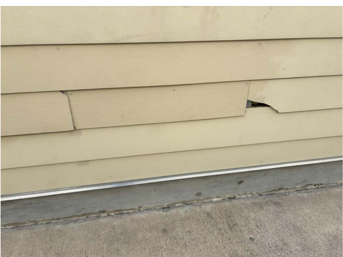
REPLACED DAMAGED SIDING
