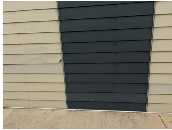
REPLACE DAMAGED SIDING
