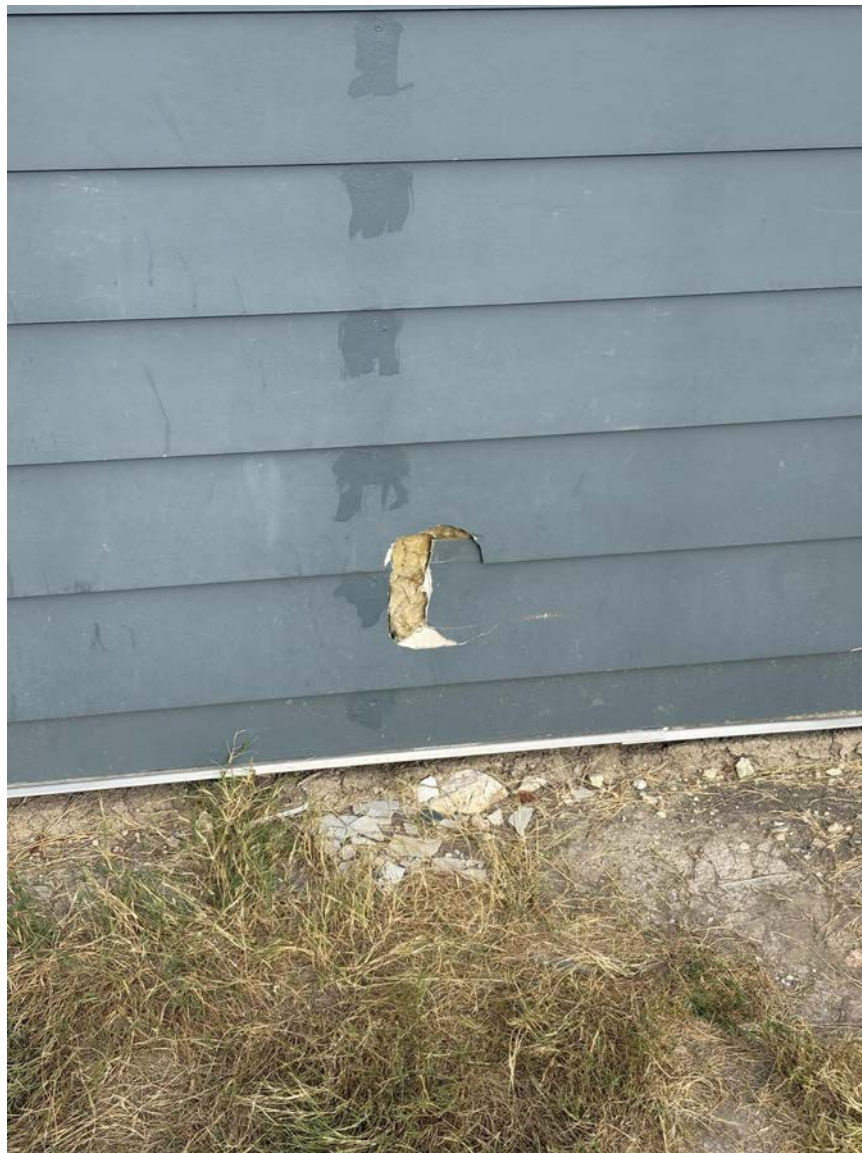
REPLACED DAMAGED SIDING
