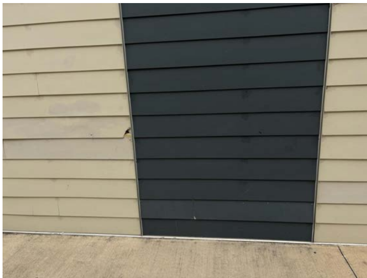
REPLACE DAMAGED SIDING
