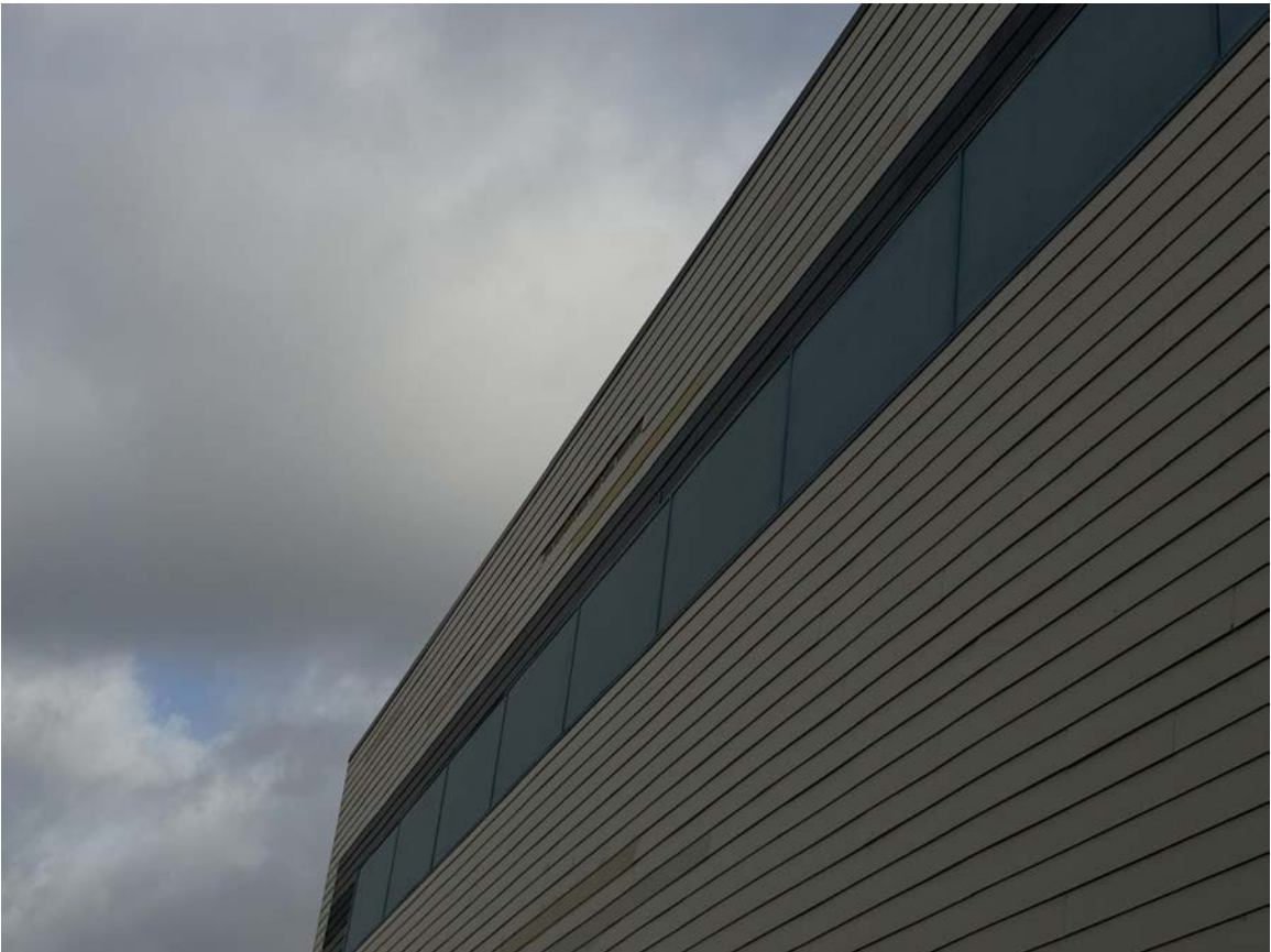
REPLACED DAMAGED AND MISSING SIDING
