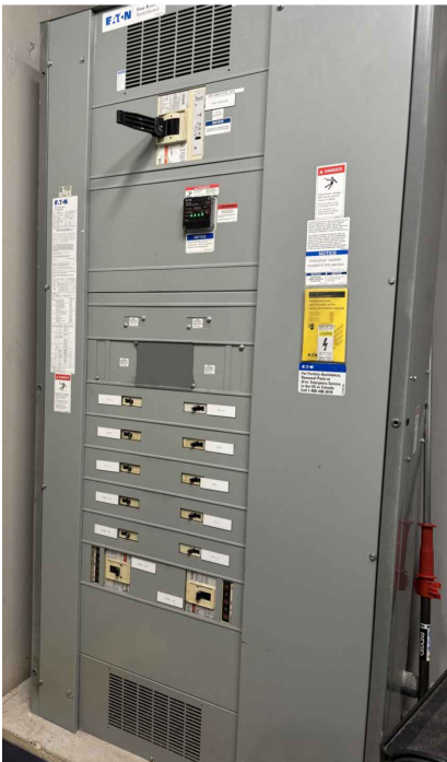
03 SWITCHBOARD "DPA" IMAGE SCALE : NOT TO SCALE.
