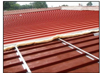
ROOF HUGGER Sub-purlin for existing Vertical Rib standing seam panels with new Trapezoidal Rib SSR.
