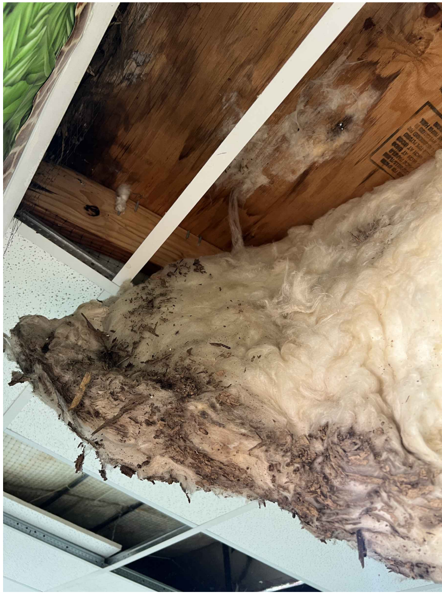
04 DAMAGE AT ROOF SHEATHING/INSUL. SCALE: NTS
