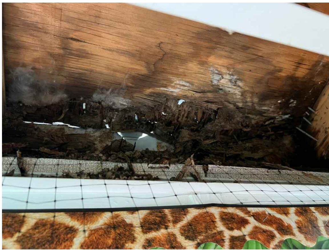
02 DAMAGE AT TOP PLATE SCALE: NTS
