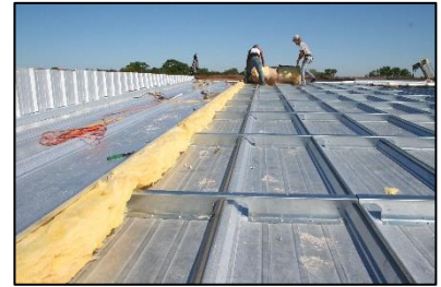
ROOF HUGGER Sub-purlin for existing Trapezoidal Rib standing seam panels with new Trapezoidal Rib SSR.
