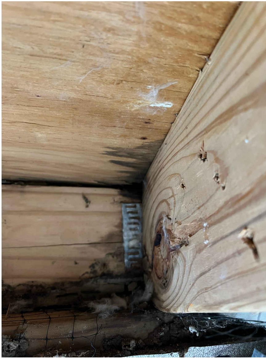
03 DAMAGE AT RAFTER TO LEDGER SCALE: NTS
