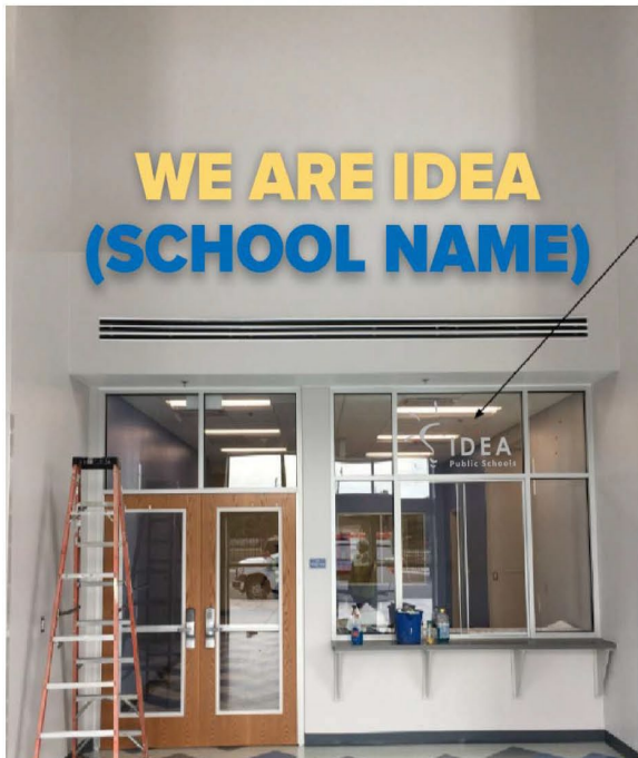
INTERIOR LOBBY WALL
