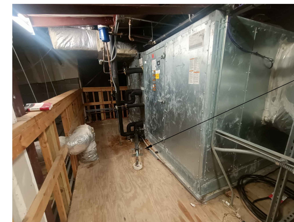
03 IDEA FRONTIER EXISTING CONDITIONS (BUILDING B - MEZZANINE) SCALE : NOT TO SCALE
