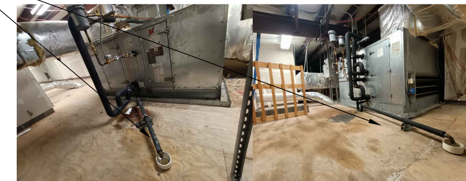
IDEA FRONTIER 03 EXISTING CONDITIONS AHU-3&4 (BUILDING C - MEZZANINE) SCALE: NOT TO SCALE
