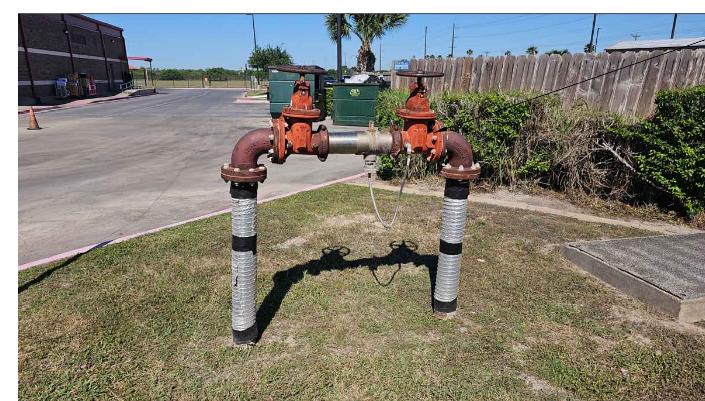
02 IDEA FRONTIER DOMESTIC COLD WATER BACK-FLOW PREVENTER (ALTERNATE #1) SCALE : NOT TO SCALE
