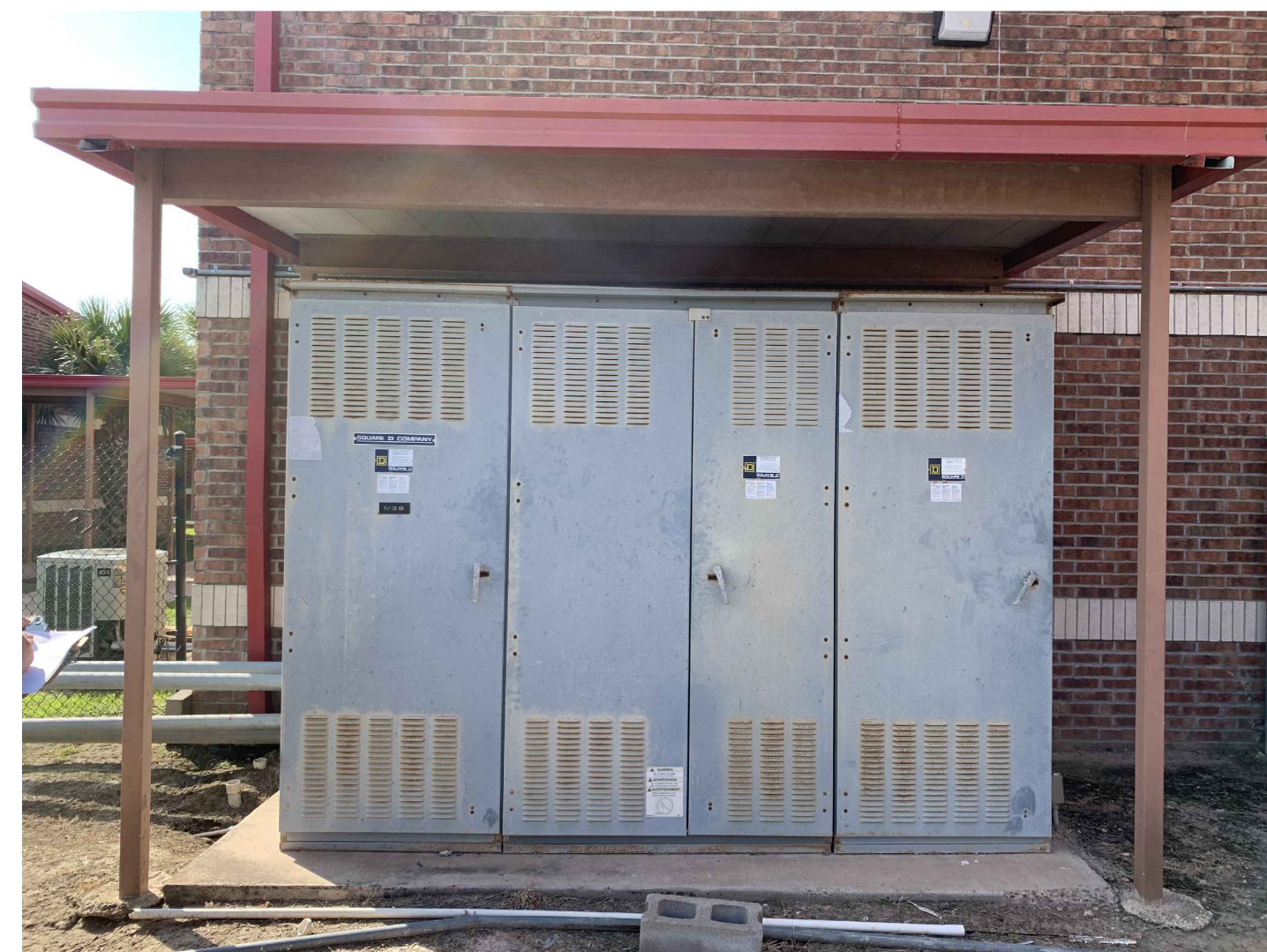
04 EXISTING ELECTRICAL SERVICE ENTRANCE SCALE : NOT TO SCALE
