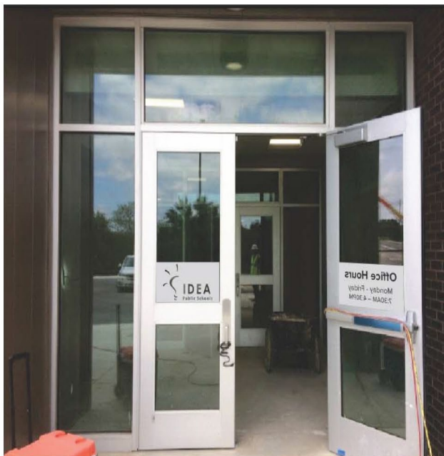
TYPICAL EXTERIOR DOORS
